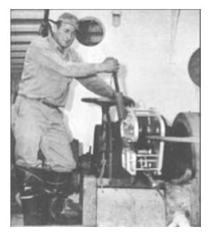
When trawling, a pair of 750-N Meters enables the winch men to accurately synchronize their winches and make corrective changes of warp settings. Meters avoid errors caused by warps stretching in service. This is particularly important during mid-water trawling. Avoid costly trips to port for remarking damaged cables.
